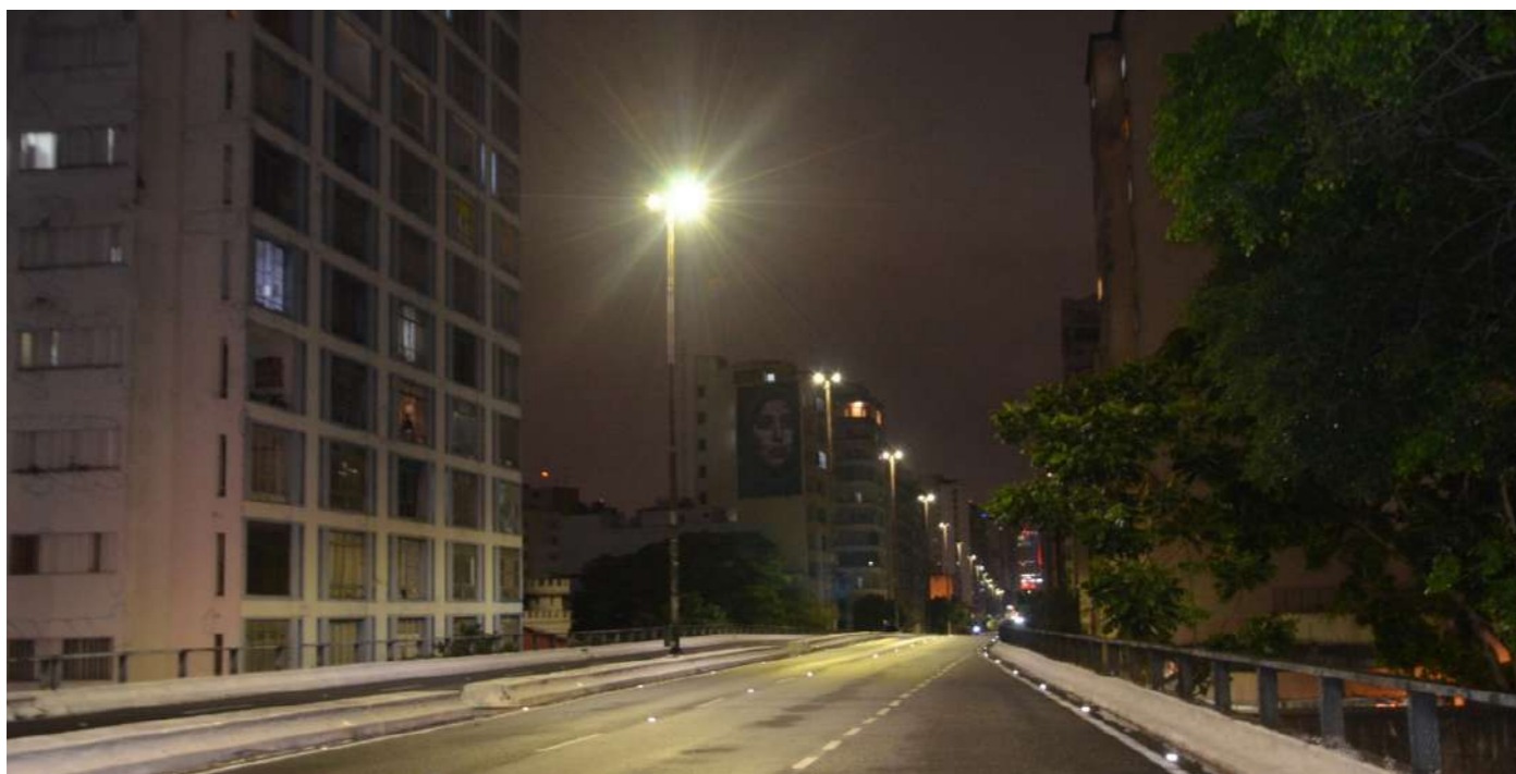
Installation of LED lights on street lamps in São Paulo.
