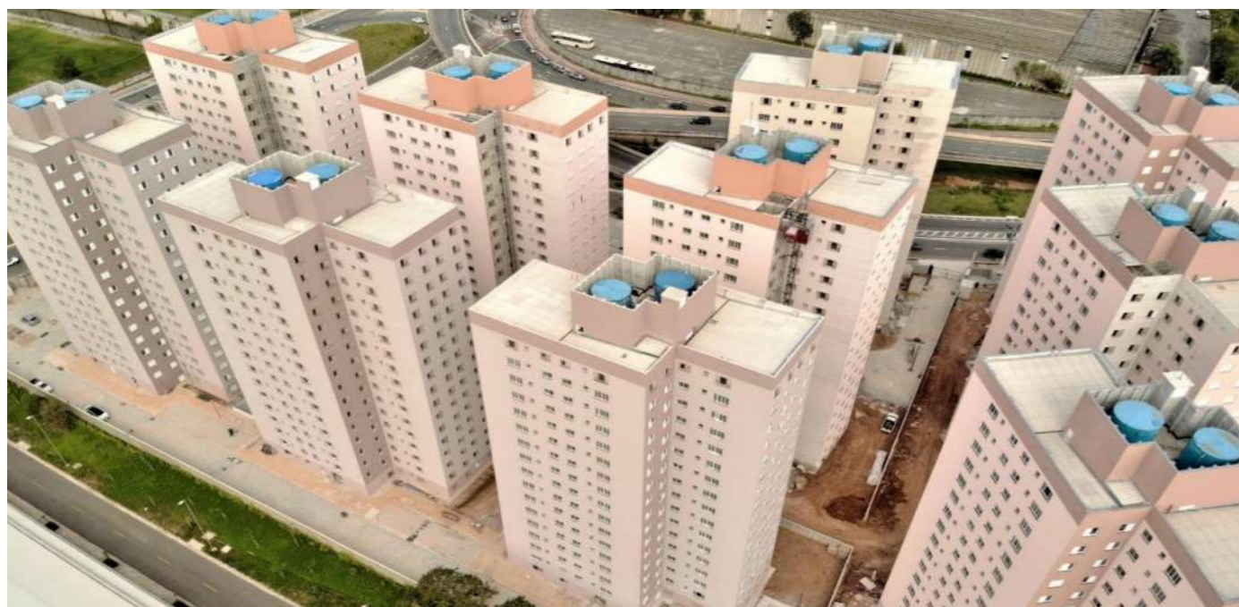
Guido Caloi Housing Units in the South Zone of São Paulo.
