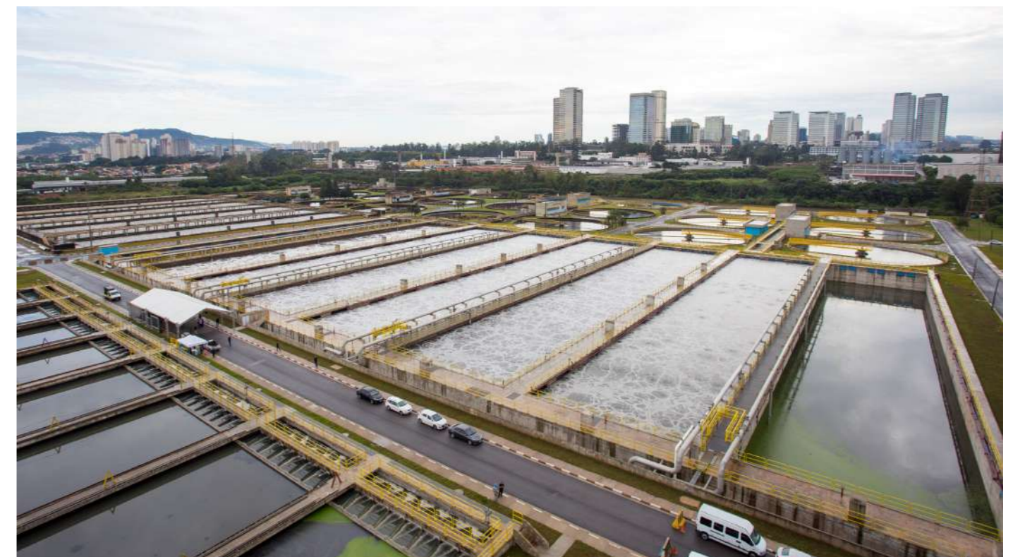
Piqueri Sewage Pumping Station.
